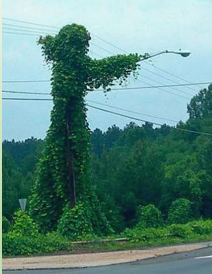
Kudzu smothering a utility pole
